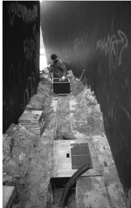
Figure 5. Installation works in March 2001.
