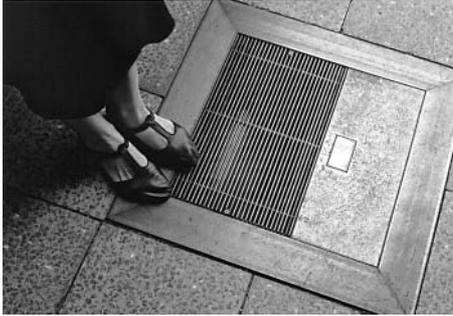
**Figure 2.** One of four ground grids with a loudspeaker and a light underneath the ground on the left side and two infrared distance sensors at the right side covered by a little window. Each loudspeaker cavity contains two sensors aimed in different directions.
